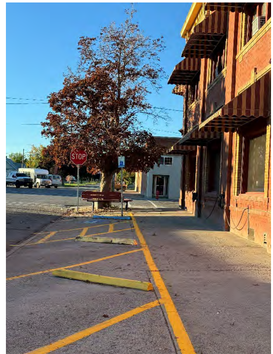
East Side City Hall looking south to Main Street
